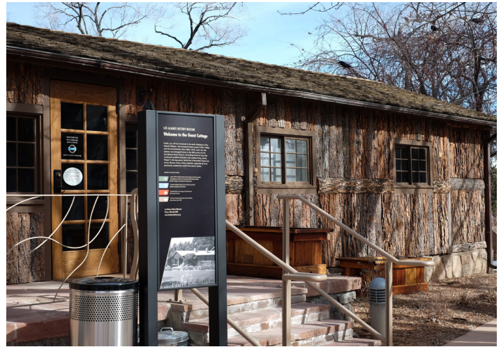
The newly renovated Los Alamos History Museum
